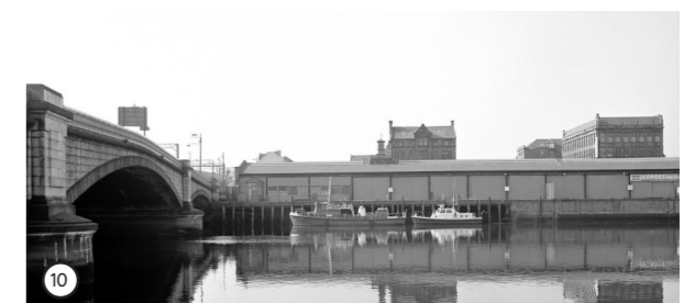
10 - Goods Shed at Clydes Place Quay - Now Demolished
