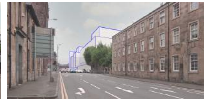
View from Cook Street
