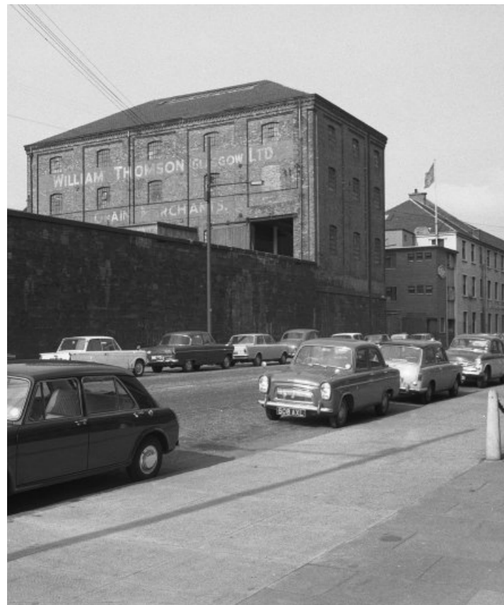
1968 Stables and Grain Merchant Building with Engine Works in background (Canmore)
