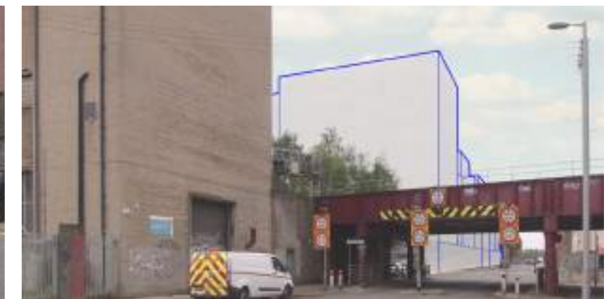
View from Cook Street
