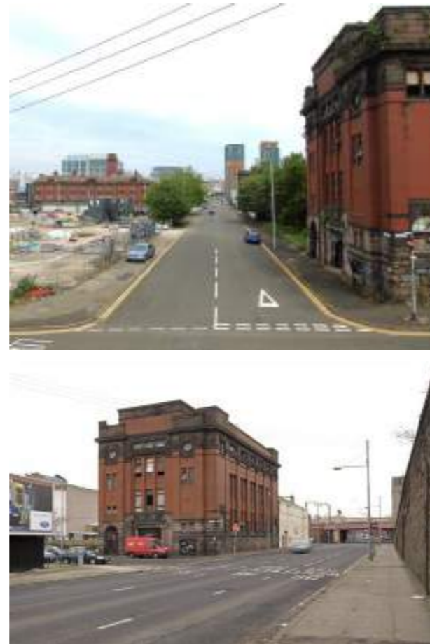
3. Former Telephone Exchange
