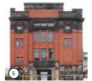
5 - Former Telephone Exchange
