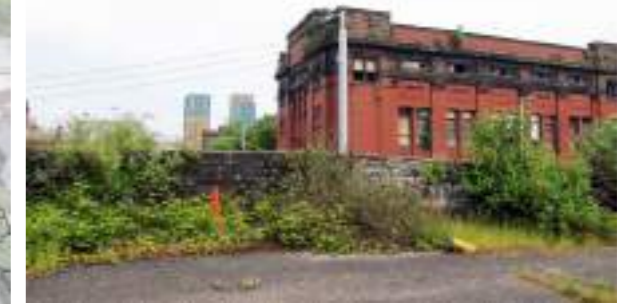
View North towards Barclays towers
