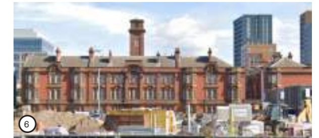
6 - Former Southern Fire Station
