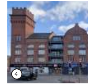
4 - Former Victoria Mills
